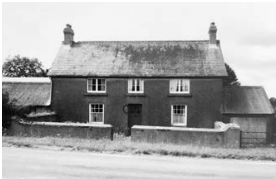
'Southfield' photographed in 1985 before total refurbishment. Courtesy of Mrs. E. Vaughan
