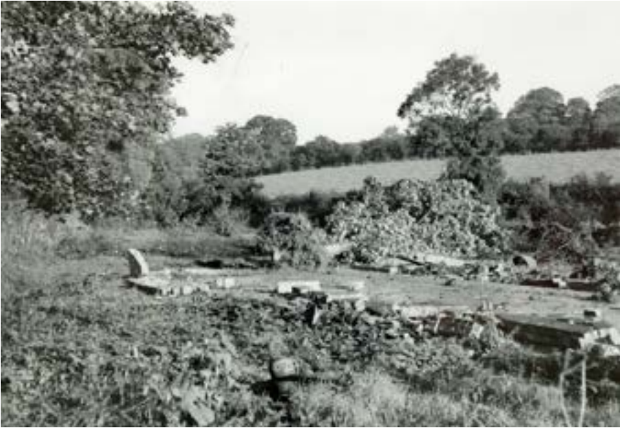
The base of the old 'New Recreation Room' during demolition in 1961
