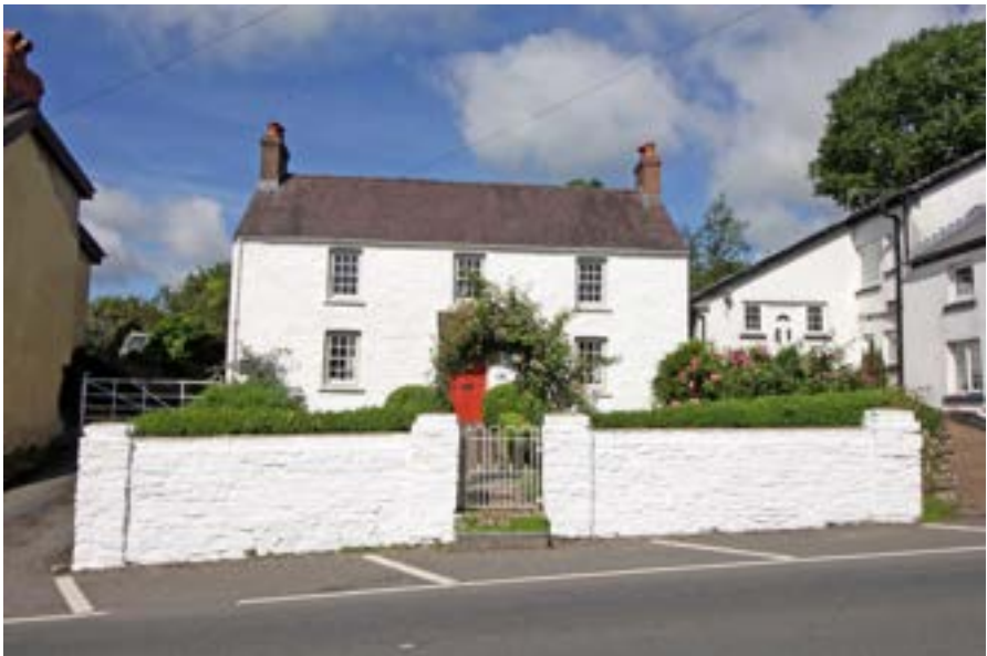
Elm Cottage following major refurbishment in 2018. All the walls have been traditionally lime-washed. To the left is 'Laburnum Cottage and the right is 'Pendre' with its 1970s extension. Photographed 2020 RLD.
