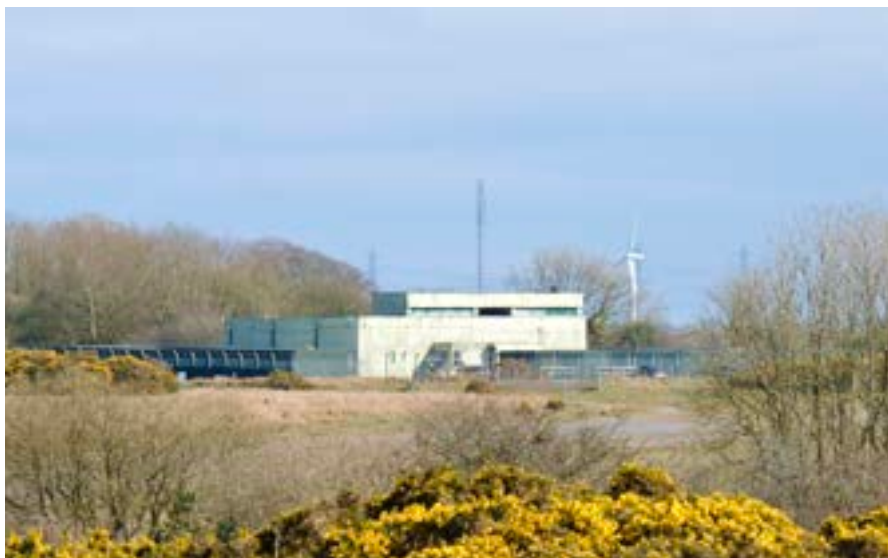
Microwave Communication Bunker photographed in 2020.
