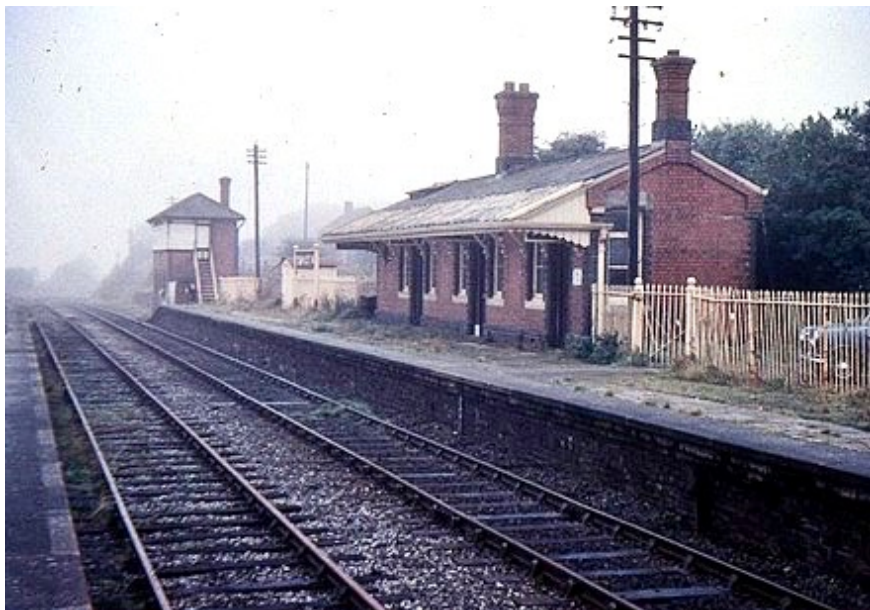
Templeton Signal Box and Station. Photographed in c.1960
